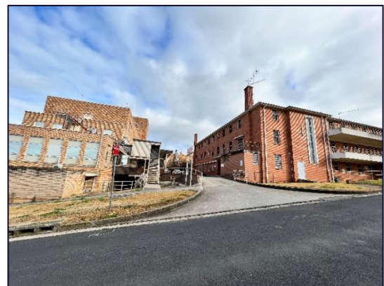
Photograph 5: View to west from Ina Drive showing terracing of the slope to accommodate footings of (a) Main hospital building (left) and 'reversed L-shaped' building (right)
